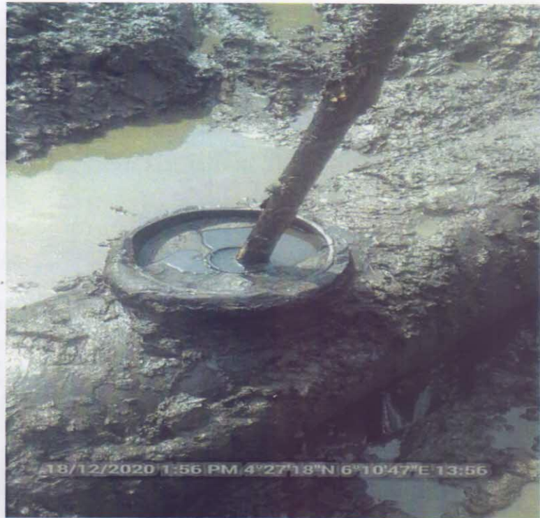
Fig B: Suspected Incident Facility shortly after excavation
